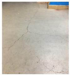
Photo 4. Cracking in floor of warehouse.
