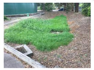
Photo 1. Stormwater retention basin.
